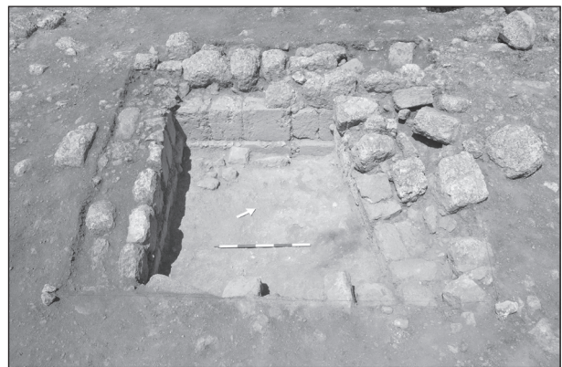
9. Trench 7: top of the make-up layer dated to the Abbasid period © LAJP.
